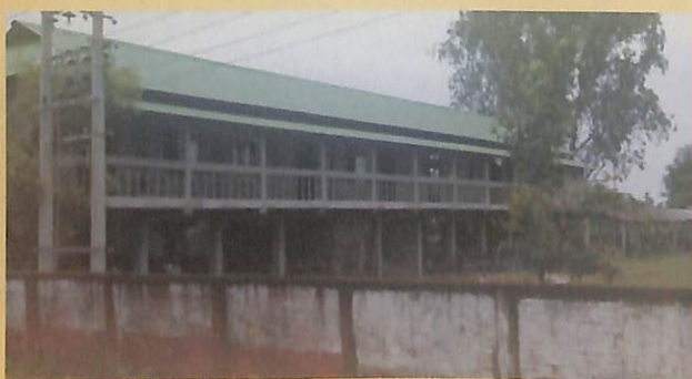
Administrative Building Under Construction
